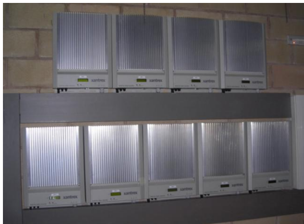
Xantrex GT5.0SP Grid Tie Solar Inverters at Premier Power solar installations in Navarra, Spain
